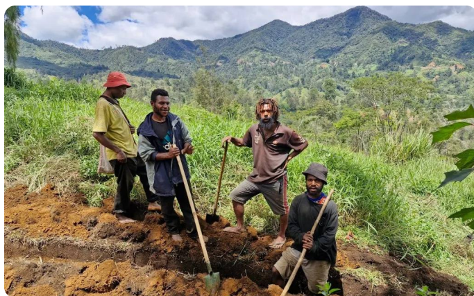
Digging the trench by hand
