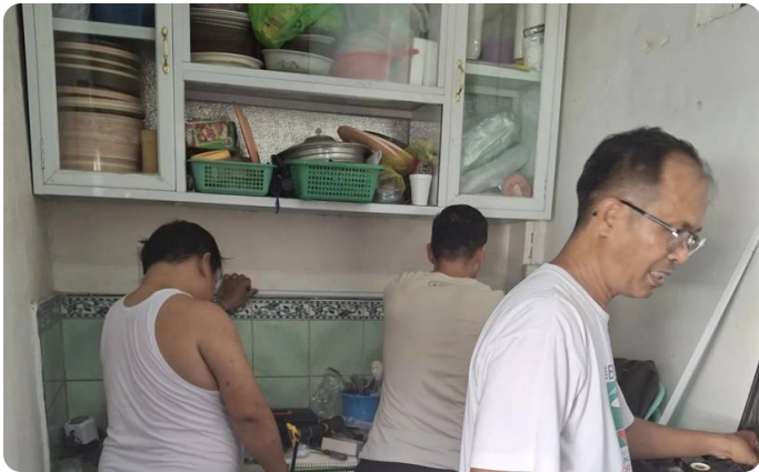
Installing the system
