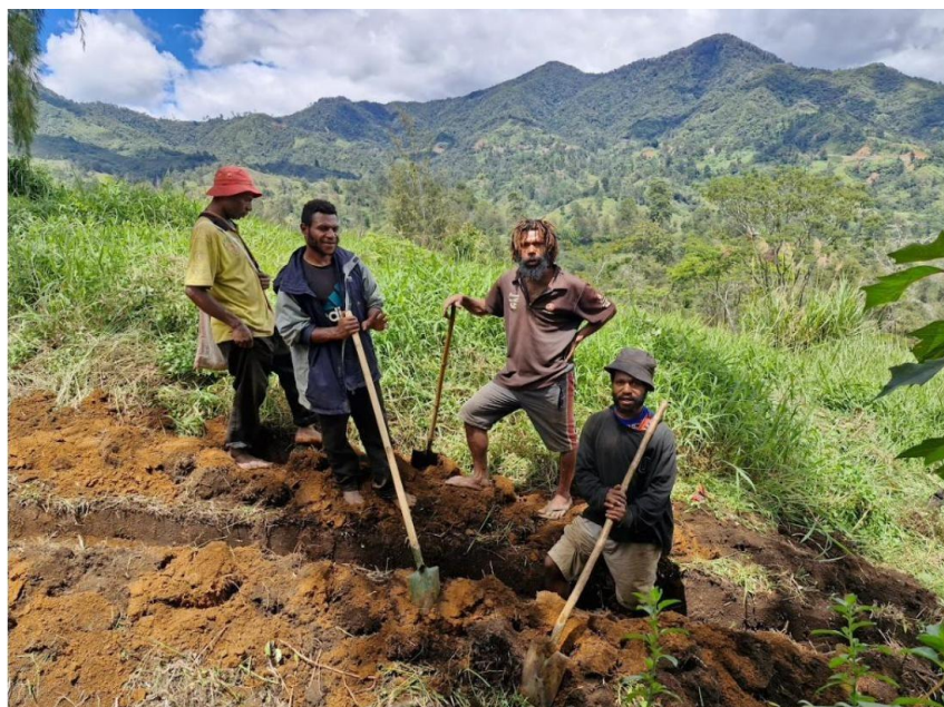
Community members hand-dig kilometers of trench up steep mountain terrain
