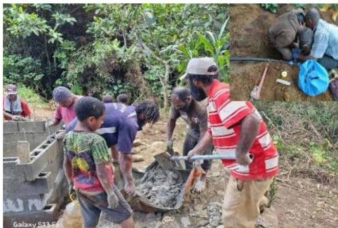
Community members mix cement for the water catchment built during Phase 1.
