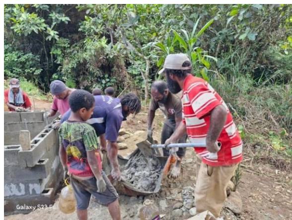
The community builds the concrete catchment by hand
